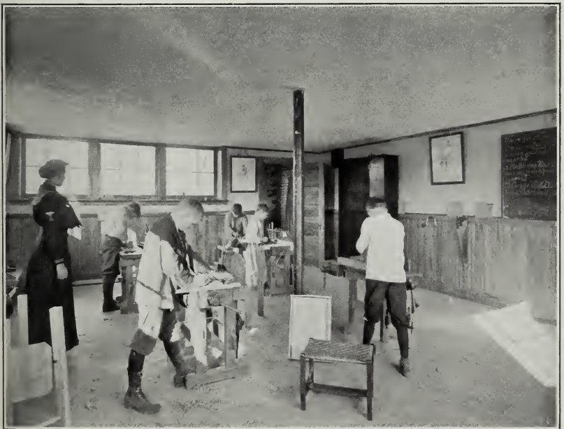
A second room in the basement of the new building at Fairmont
